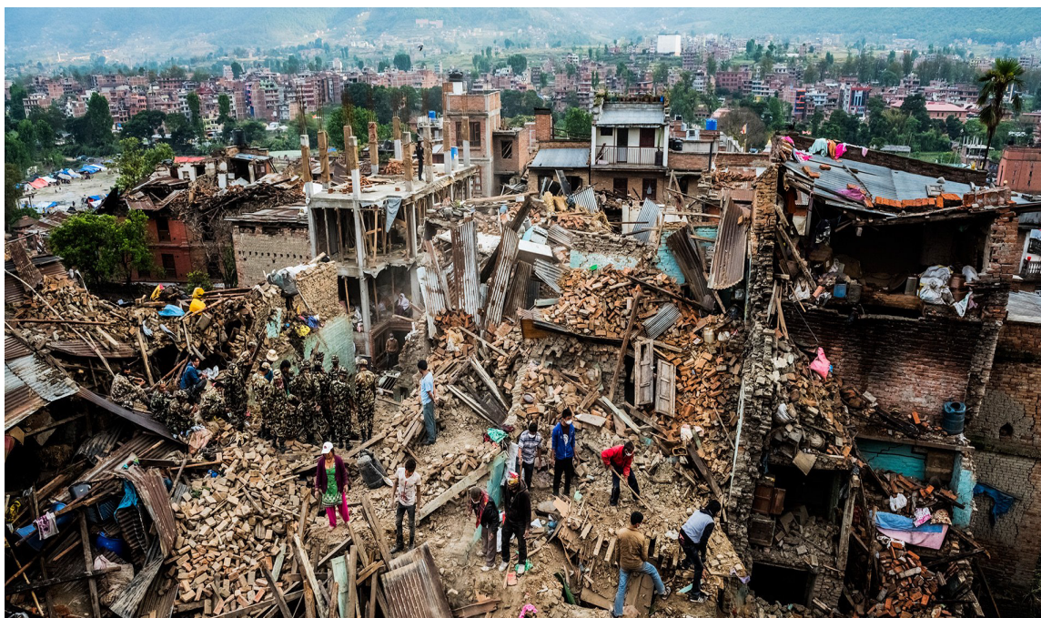
7.8 Richter scale earthquake - 2015 killed 9000 people and destroyed 80000 infrastructures generating 14 million tons of waste
